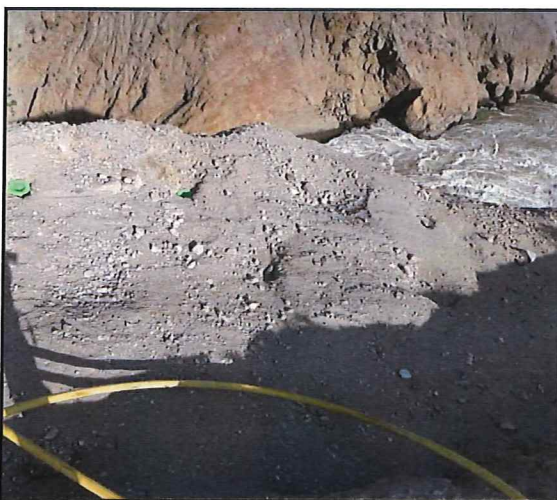
Figure 1. Holes drilled by scaling crews.
